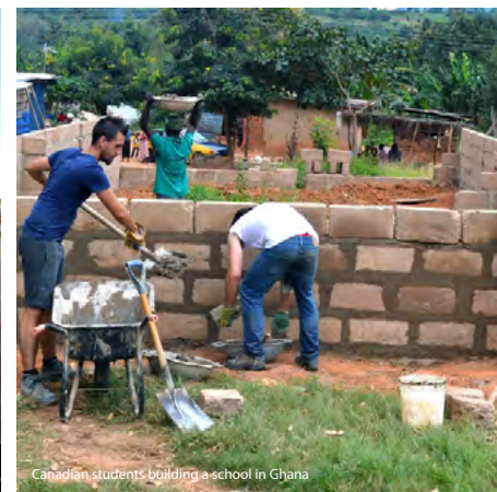
Canadian students building a school in Ghana
